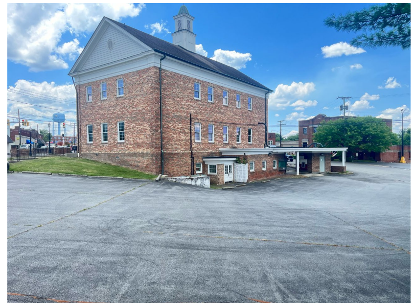
Building Side View from Upper Parking Area
