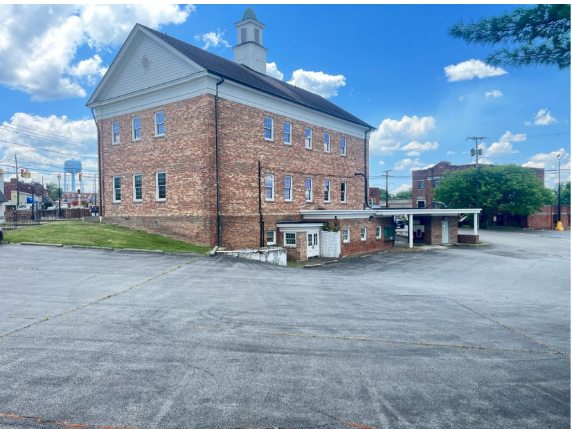
Building Side View from Upper Parking Area
