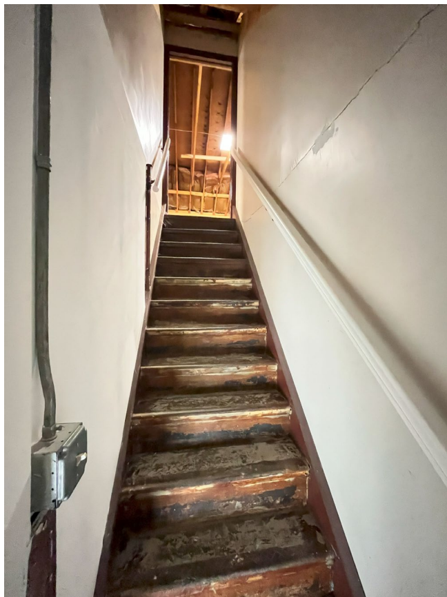
Stairway to Attic Floor
