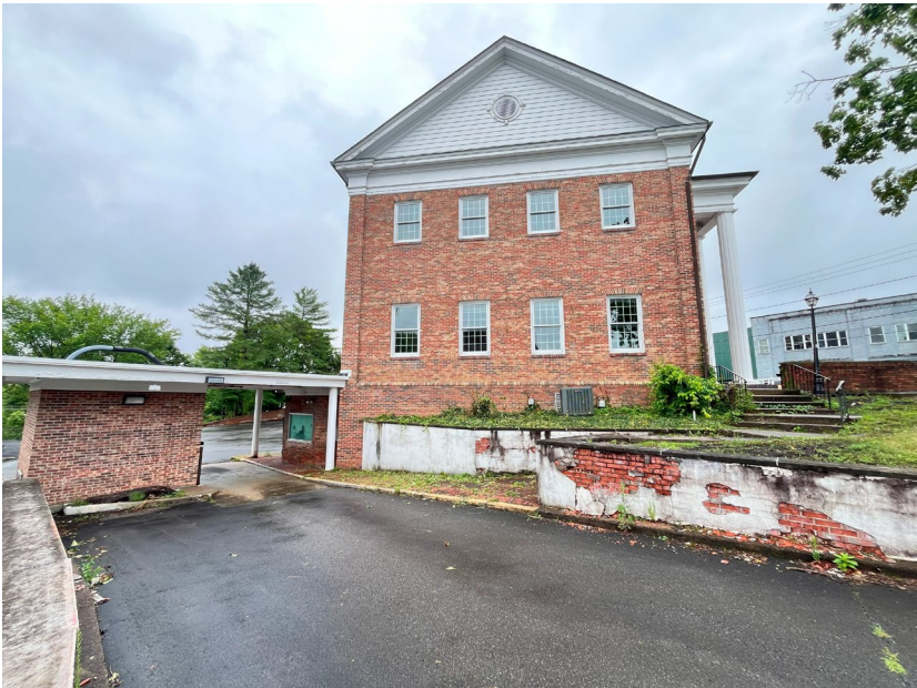
Building Side View with Drive- Through and Retaining Wall
