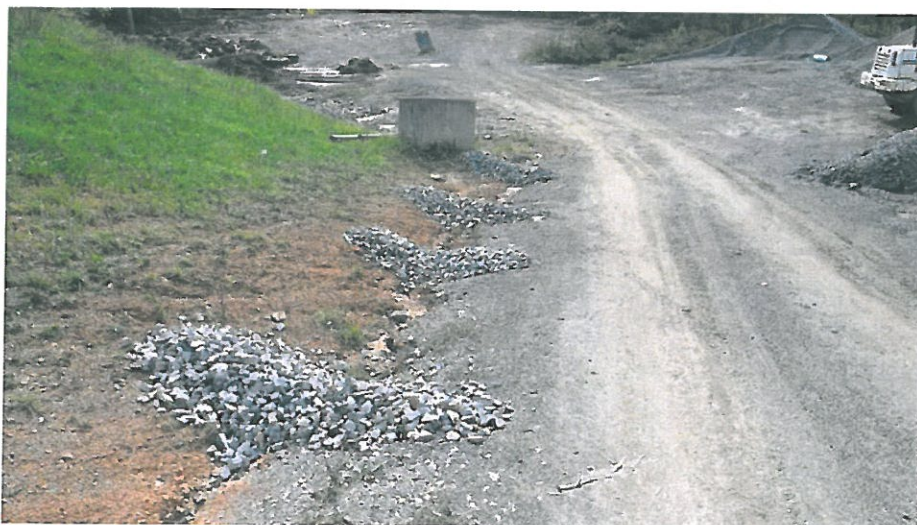
Vegetated soil with gravel water breaks to provide collection of salt shed run off.
