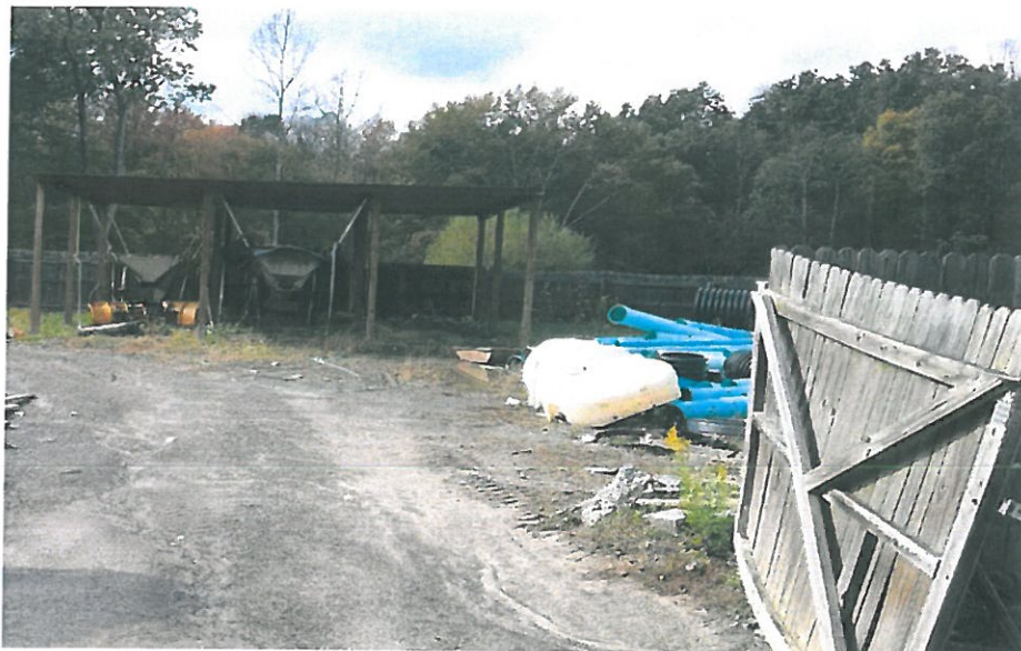
Enclosed storage area. Salt spreaders are covered and suspended.
